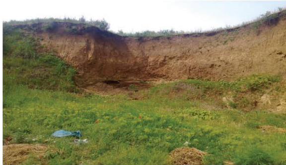
Figure 1. Collapse of shore in Fălcoiu locality
