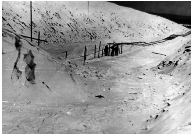
Photo 2. Mounds of heaving ground do not have considerable impacts on humans since the lands where they occur are usually sparsely inhabited and poorly developed. The photo shows mounds of heaving ground on the Tynda–Zeysk section of the Baykal—Amur Railroad, Russia (Photo credit: V.S. Afanasenko, Department of Geocryology, Moscow State University, Russia)
