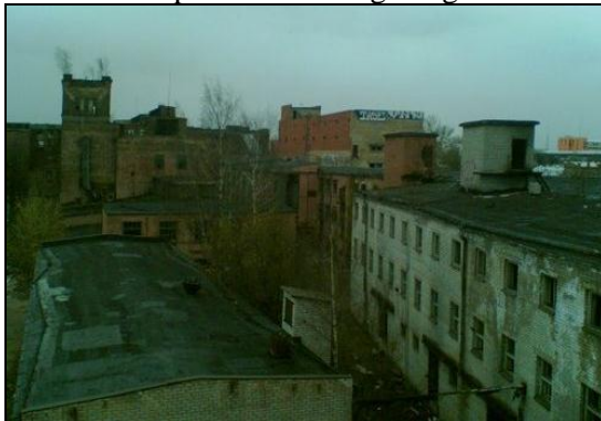
Figure 4. Abandoned bicycle and moped factory, partly demolished
